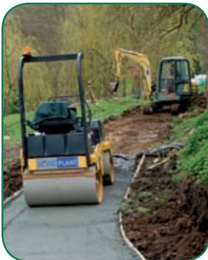
Above: Steps now lead down from the old carriage avenue. Left: Diggers excavate soil to create new paths that are then rolled level. Right: A new path leads from Cherry Tree Avenue alongside the Elizabeth Harvie field.
